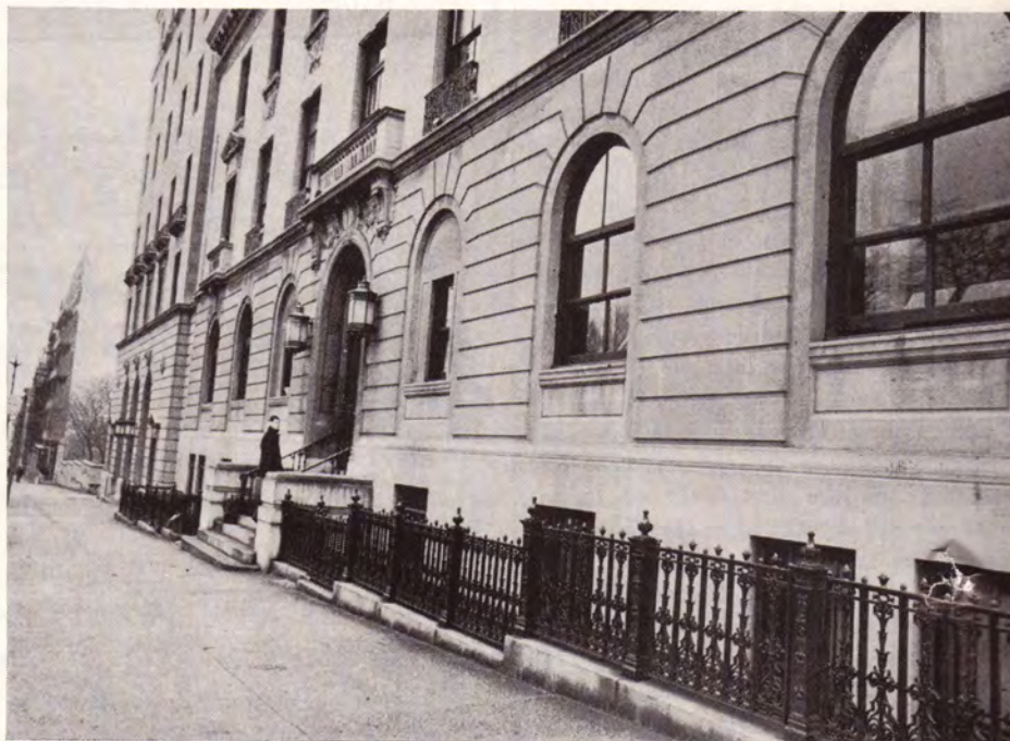
SOLID STRUCTURE: The Juilliard School of Music, on Morningside Heights, has included a dance curriculum for 11 years. The school moves to Lincoln Center in (tentatively) 1965.
